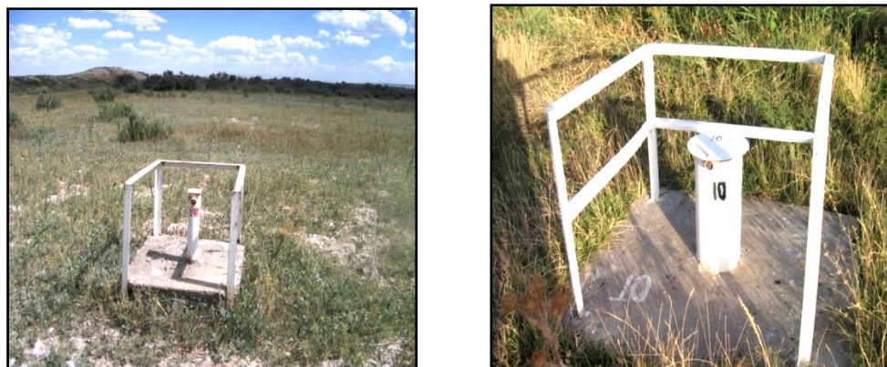
Figure 2 – Pictures of central and observation wells No. 261, 10
